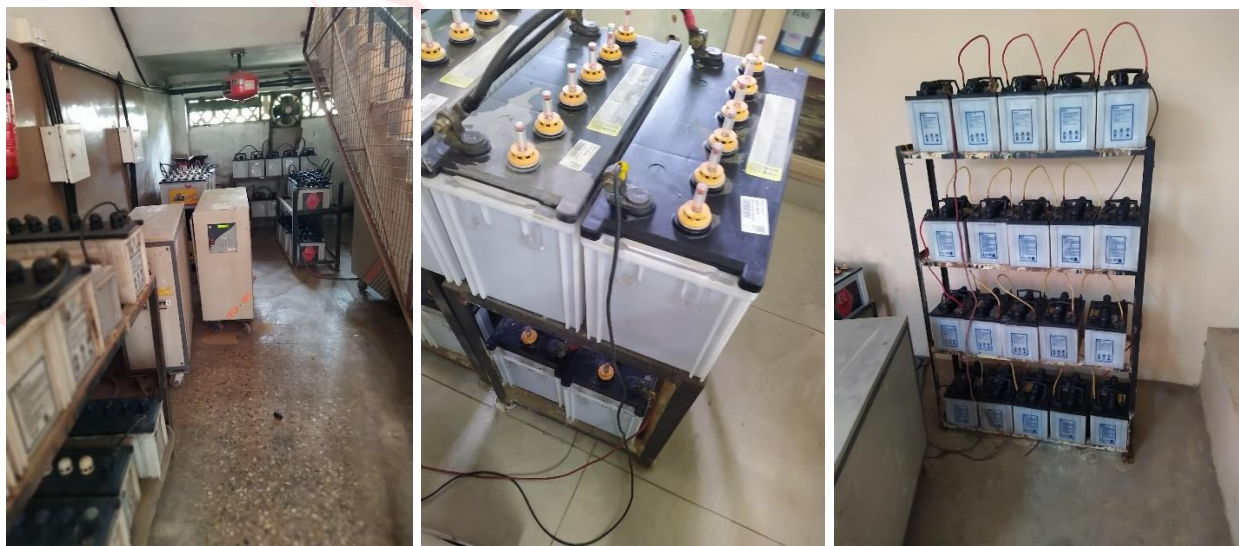
Figure 15 - Battery placement, Need cross ventilation.
