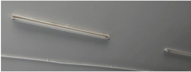
Figure 11 - T5 & T8 tube lights with Electromagnetic choke
