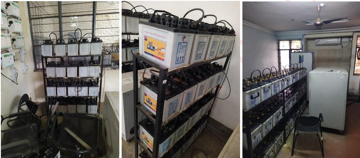
Figure 15 - Battery placement, Need cross ventilation.
