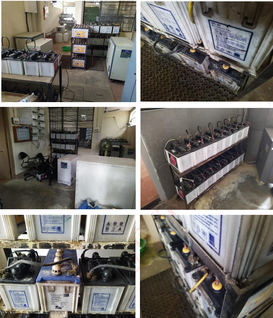
Figure 18 - Galvanic reaction causing damage to battery life
