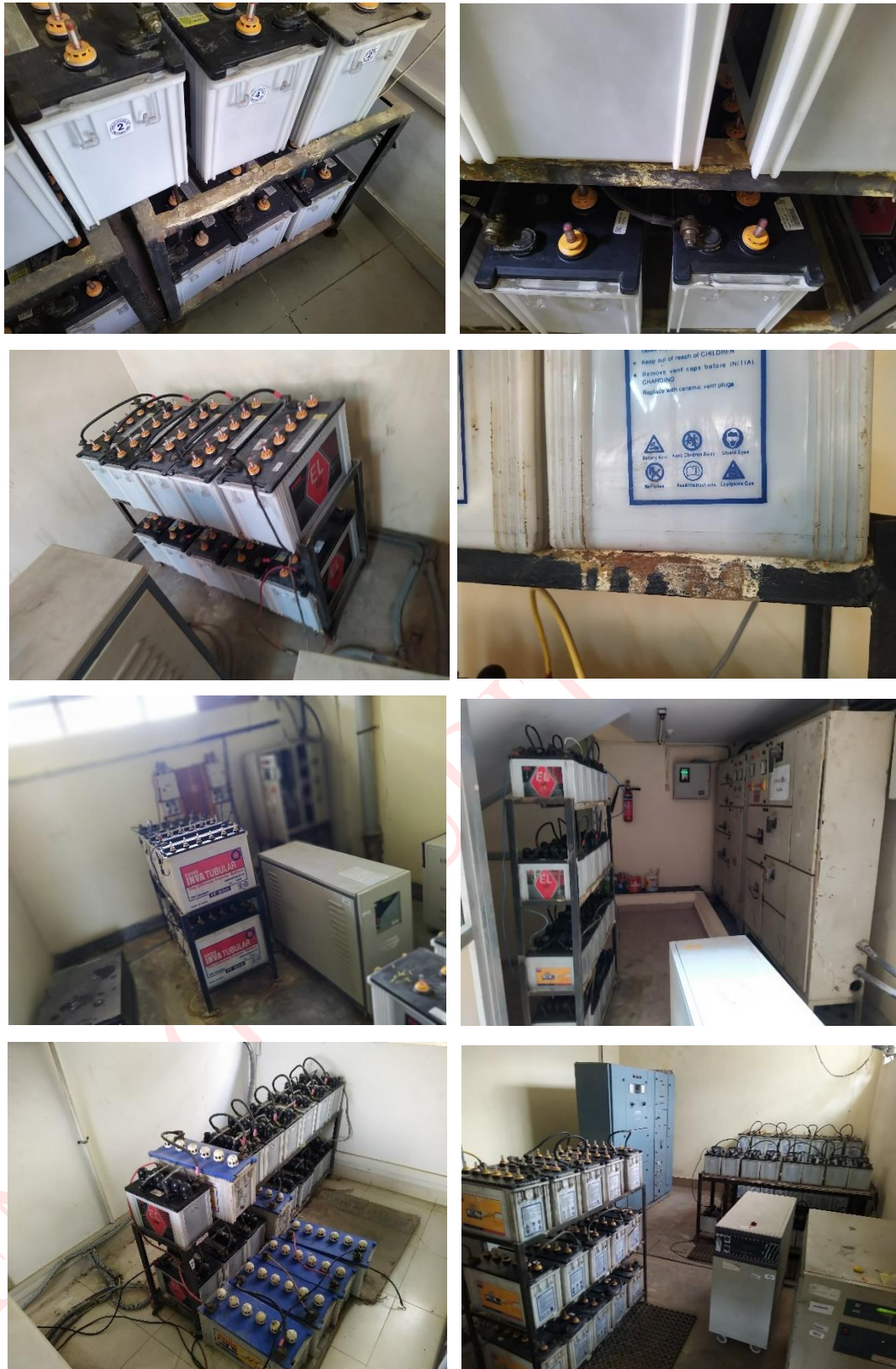
Figure 16 - Thickly populated & stacking in unventilated area
